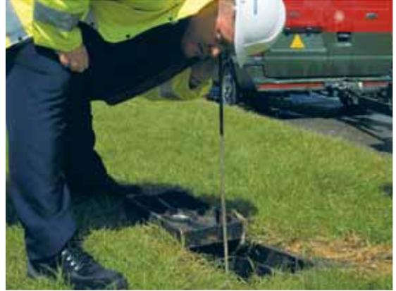
Listening for leaks; the first stage in detection and repair.
