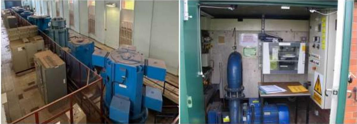
*Images above show Hampton Loade’s high lift pump hall at 12 MW of installed pumping capacity, and a small distribution booster of 30 kW capacity. Both of these sites would be treated equally in the booster stations per length of main variable, counting as one site each, which is clearly not reflective of the power costs nor the capital maintenance requirements.*
