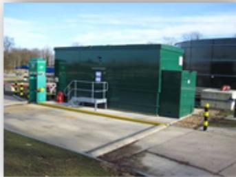
The AMP5 Standard product design has a single bunded tank arrangement with separate dosing kiosk. The product comes in 3 different tank sizes.
