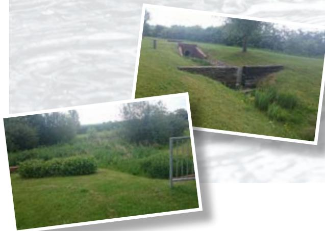
Reduces the risk of flooding and erosion by controlling flow volumes and frequency of surface water runoff
